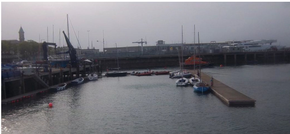
Figure 2.14: NYC Mooring pontoon
